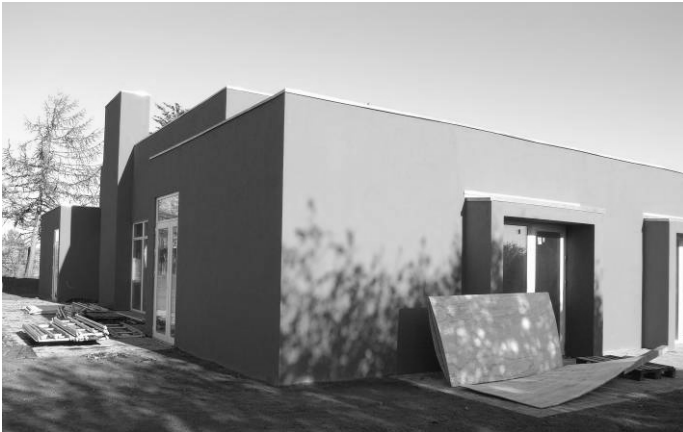
Figure 8. Photo of the centre for senior citizens – under construction.
