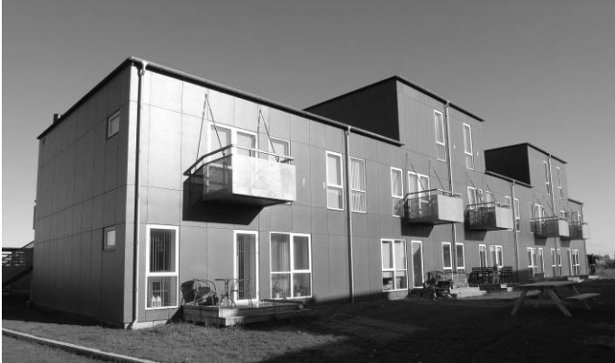
Figure 6. Photo of the KAB-ultralow-energy housing project.
